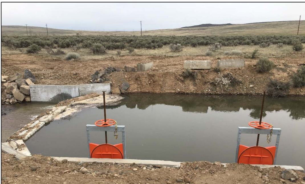
Figure 2. BLM Pit check structure and headgates on Canyon creek
