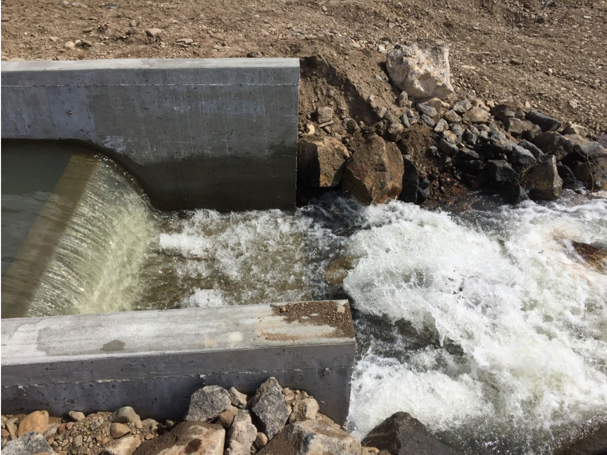
Figure 5. Measurement weir for recharge inflow to the BLM gravel pit
