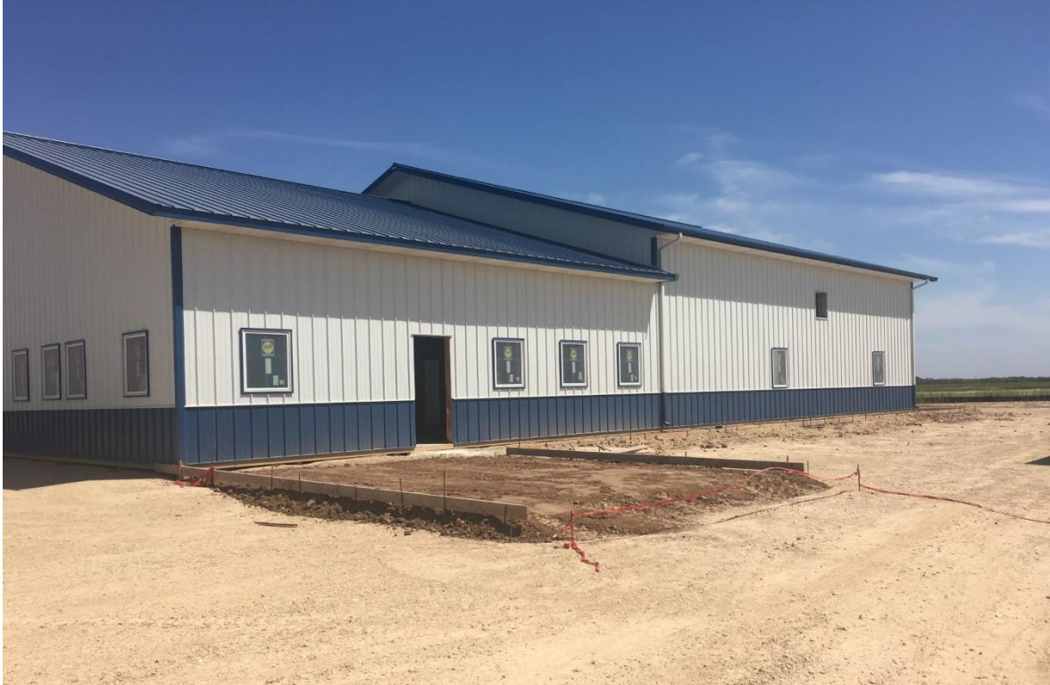
Image 1: Typical O&M Building
