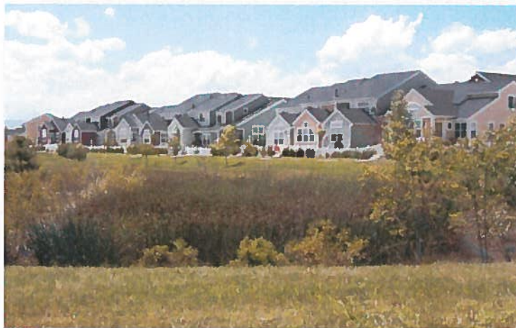
Landscaped Retention Basins
