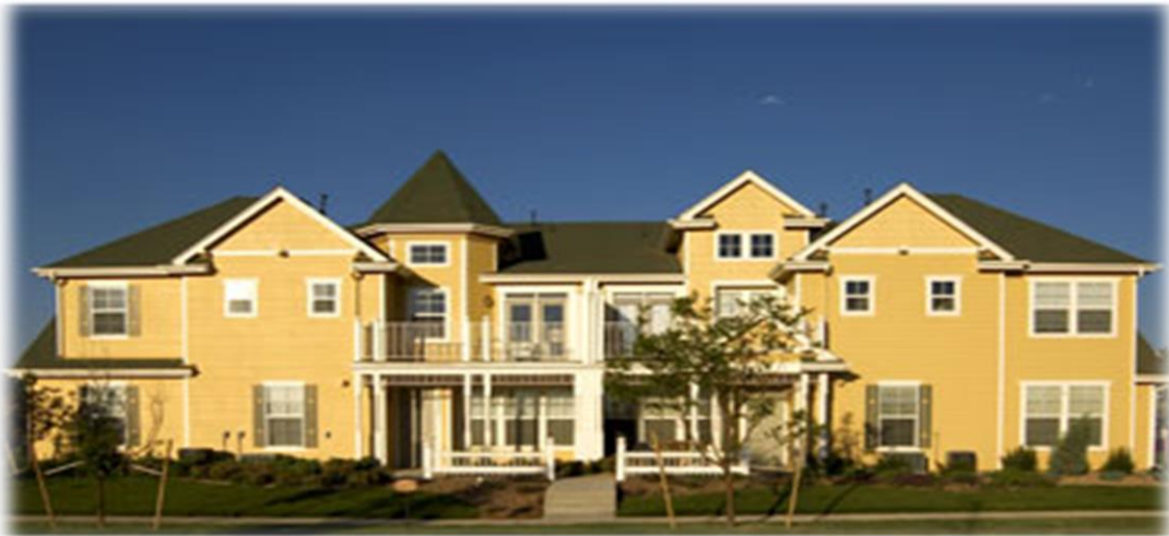
Example of multi-family dwelling with modulated facades, varied roofs and prominent entryways. Also highlights appropriate placement and percentage of windows.
