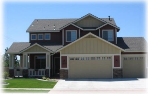
Example of Mid-Block Lot with Front Loaded Modulated Garages
