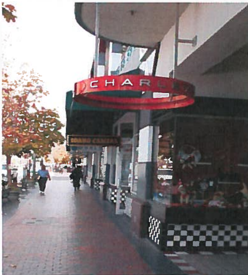
Larger Windows with Kick Plates and a Brick Paved Sidewalk
