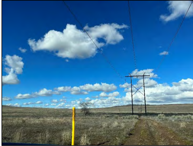
Photo 16. Transmission lines and natural gas pipeline connection, view facing north.
