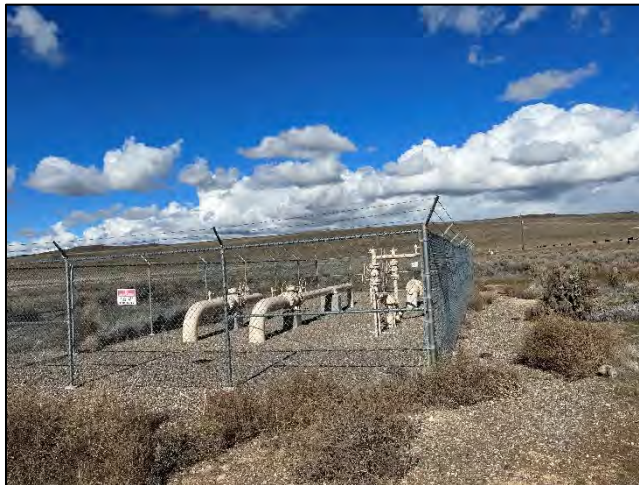
Photo 17. Natural gas pipeline access area, view facing north.
