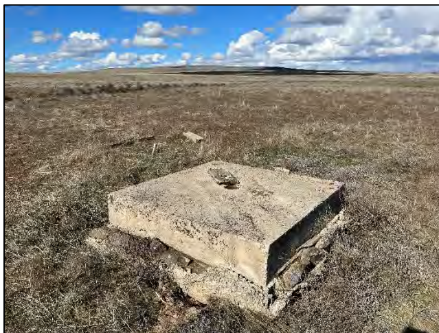
Photo 9. Abandoned cistern in the southwest of the subject property.
