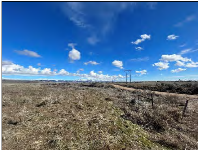
Photo 2. View of the powerlines and access road on south of subject property, facing east.
