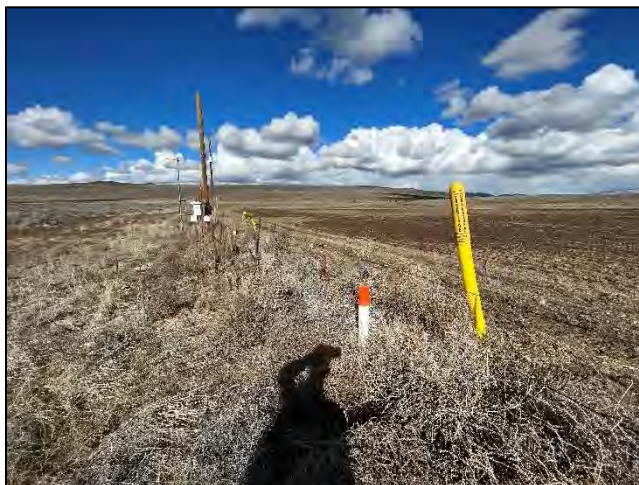
Photo 18. Natural gas pipeline, view facing north.
