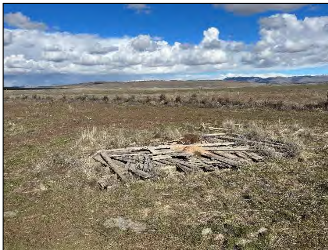
Photo 11. Building debris in the southwest portion of the subject property.
