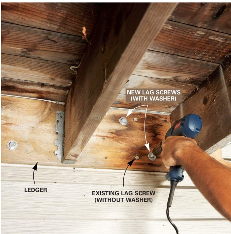
FIGURE 14: ATTACHMENT OF LEDGER BOARD-TO-BAND BOARD
