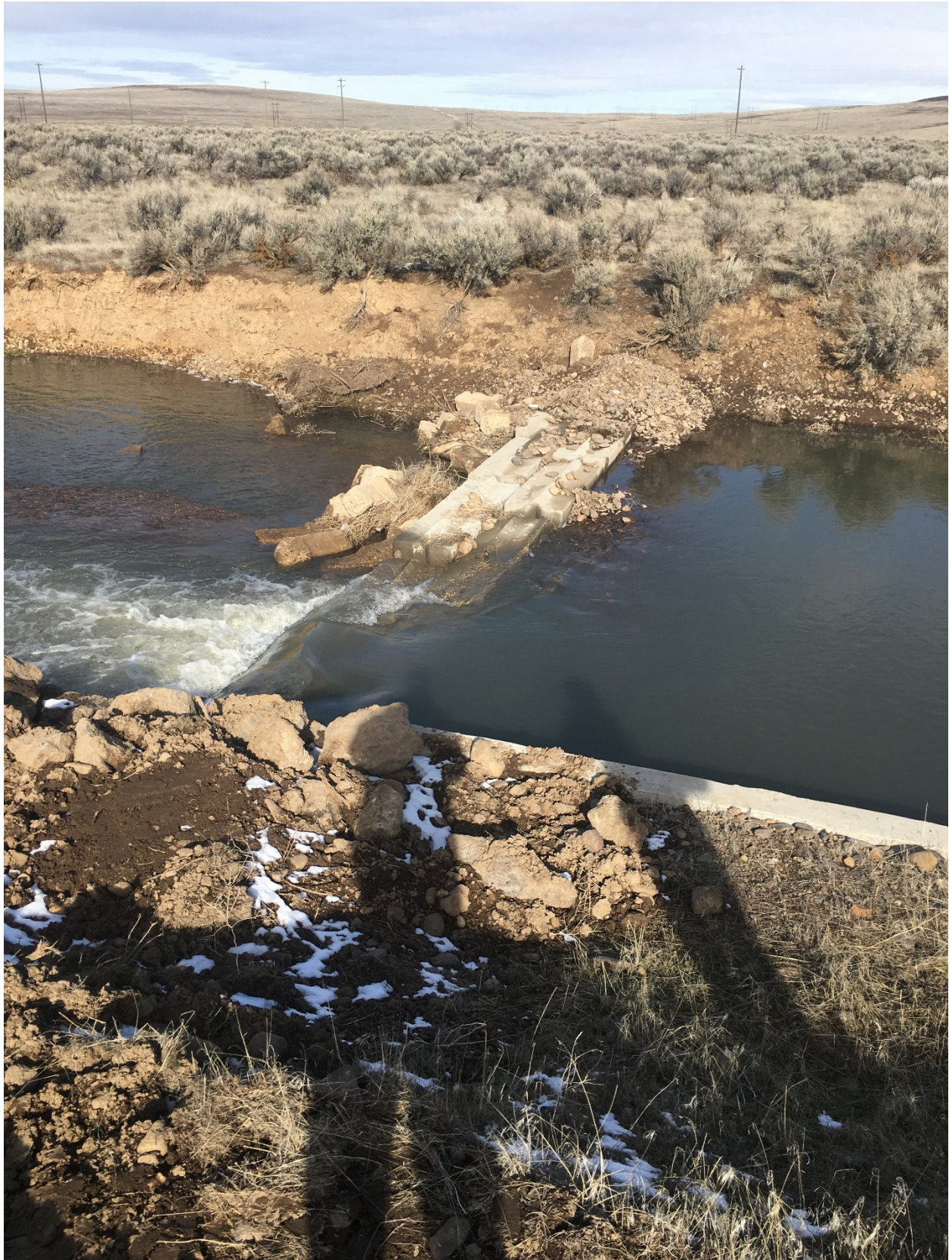
Photo 5. Check dam at Canyon Creek diversion. Photo taken on 3/1/2017.
