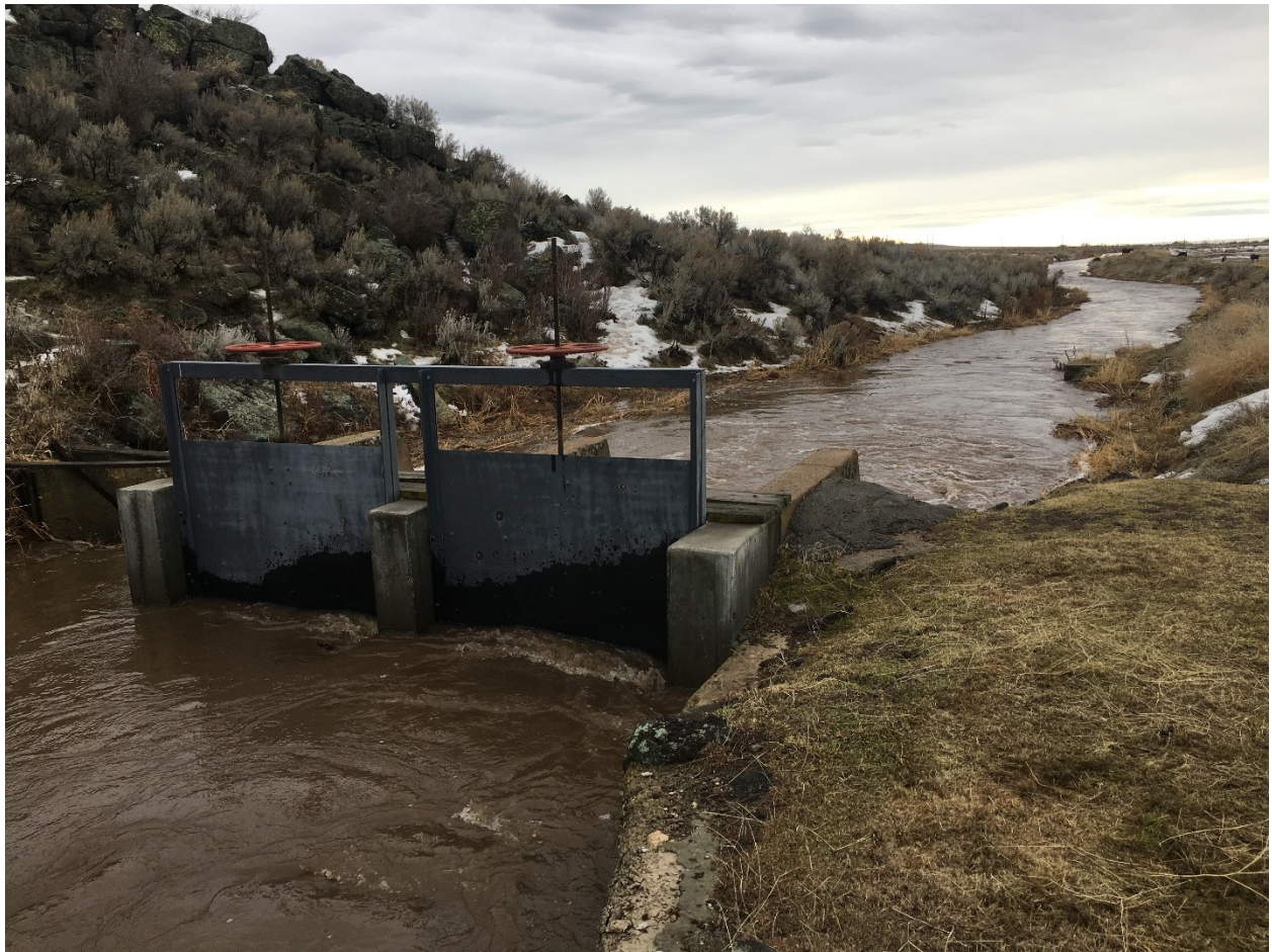
Photo 2. Head gate structure on the Mountain Home Canal. Photo taken on 2/9/2017.
