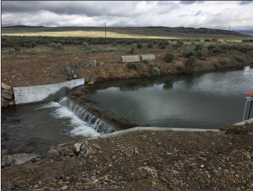
Figure 3. Check structure on Canyon Creek at BLM Pit. Removable ecology blocks are placed on concrete sill to raise the water level at the headgates.
