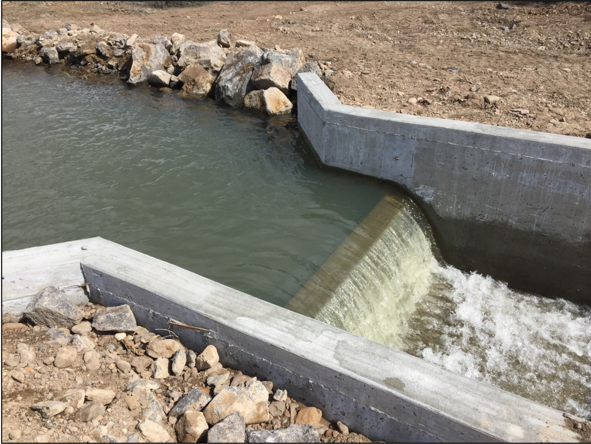
Figure 5. 8-foot suppressed weir at BLM Pit
